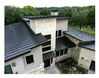
APEX Roofing was able to complete the job in just four days, overcoming challenges presented by the low slope of the roof by adding winter guard underlayment. They also provided quality installation expertise that will aid in the ongoing performance and reliability of the roof, such as changing it from non-straited to straited to help protect against regional climate conditions.
